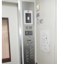
Elevator repair work
