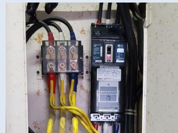
Installed electronic breaker (Artiza Kamimaezu) (Artiza Sobudai)
