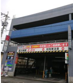
Painting work on exterior wall of parking
