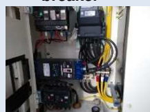
Electronic breaker installation (Installed at 12 properties)
