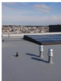
Rooftop waterproofing work
