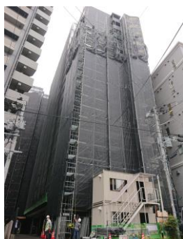
Exterior wall tile repair work
