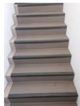
New establishment of flooring for stairs
