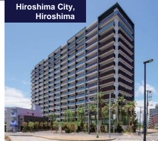
■ Polestar Ujina Kaigan Harbor View
