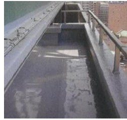
Rooftop waterproofing work
