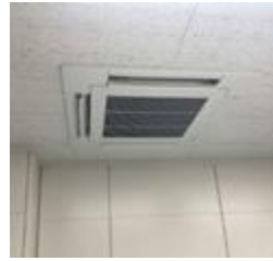
Renewal work of air conditioner
