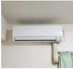
Exchange of air conditioner
