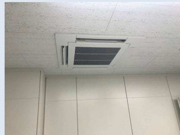
MRR Delta Building (exchanged air conditioners)
