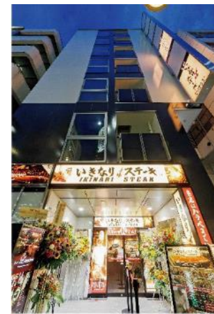
M Building Ebisu I
