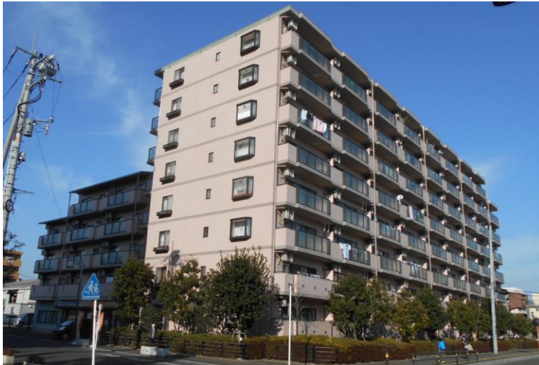
Exterior (repair of tiles, etc.)
