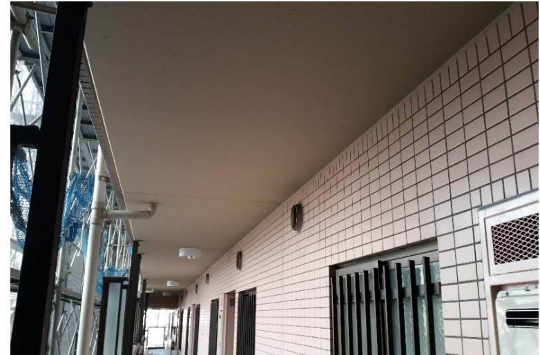
Outside corridors (repair of ceiling over corridors)
