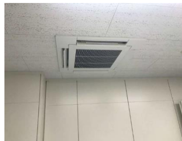
Replacement of air-conditioning system (MRR Delta Building)
