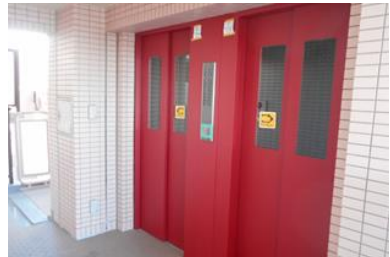
Elevators (repair of exterior)
