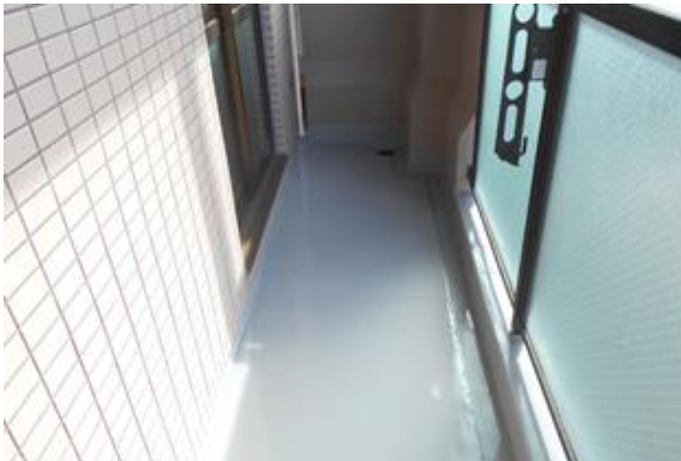
Veranda (repair of walls, repair of waterproof urethane floor *For repairing walls, dirt-proof coating was applied.
