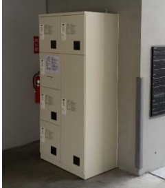
Installation of delivery box
