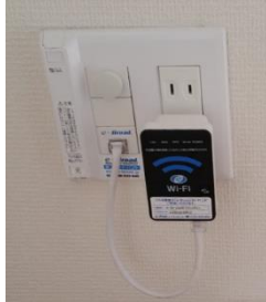
Installation of free internet (Wi-Fi)
