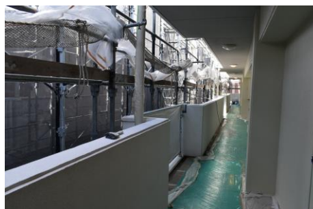
New installation work for long sheets
