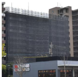
Anti-stripping agent coating work
