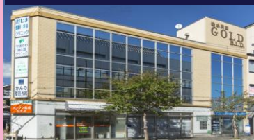
Tariumekimae Gold Building
