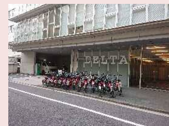
Bicycle sharing installation (MRR Delta Building, etc.)
