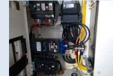
Electronic breaker installation (Installed at 13 properties)
