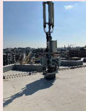
Installation of base stations of mobile phones, etc. (Artiza Kawasaki East)
