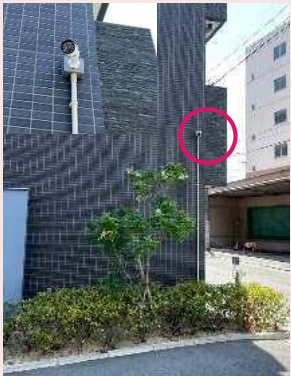
Security camera installation (Artiza Awajeki-higashi, etc.)
