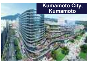
● The Kumamoto Gardens Kumamoto City's Sakuramachi District Class 1 Urban Area Redevelopment Project * Residential building
