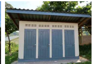
Toilet construction costs
