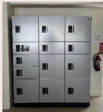
Delivery box installation (Artiza Higashi-Betsuin, etc.)
