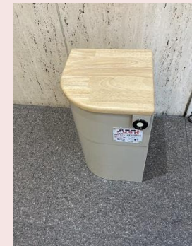
Installation of disaster prevention equipment in elevators (Ikeshita ES Building)
