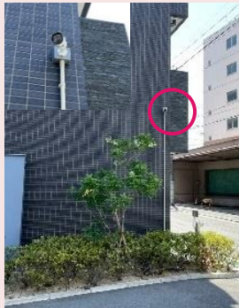
Security camera installation (Artiza Awajeki-higashi, etc.)
