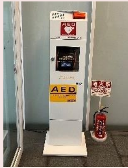
AED installation (MRR Delta Building, etc.)
